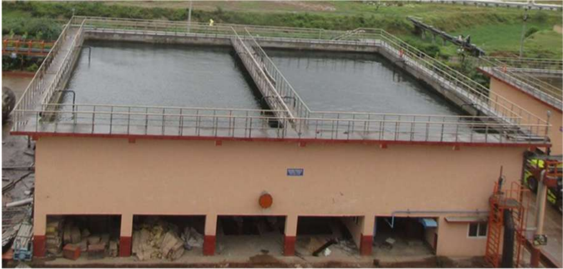
Fig.2.10: Guard ponds for storage of treated Effluent
