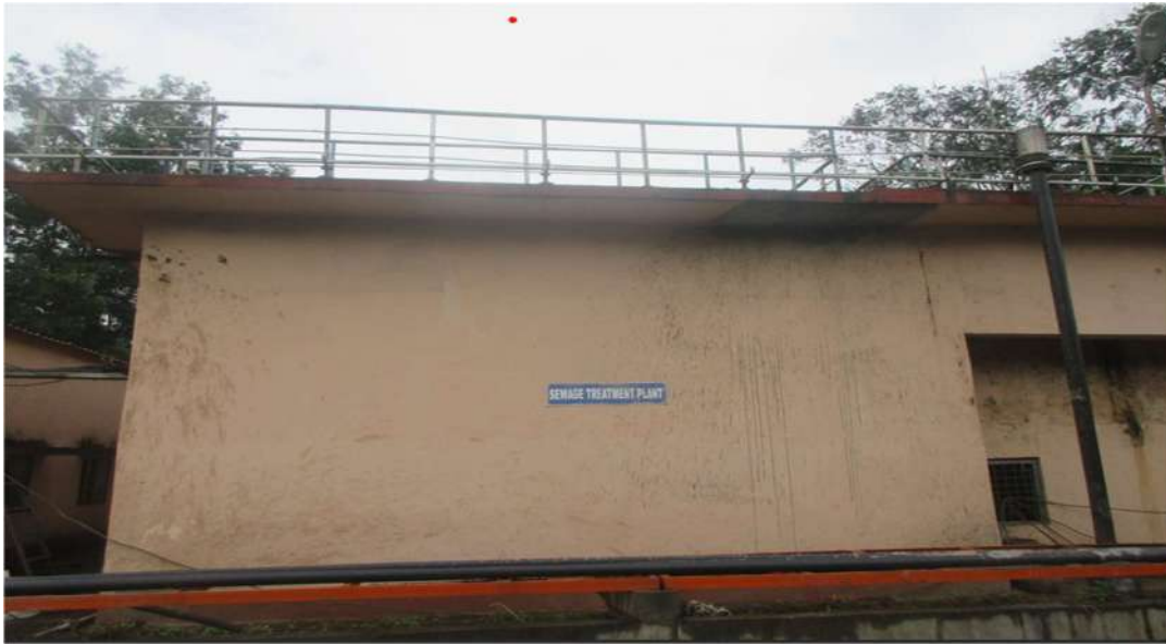
Fig.2.6: Sewage Treatment Plant (STP)
