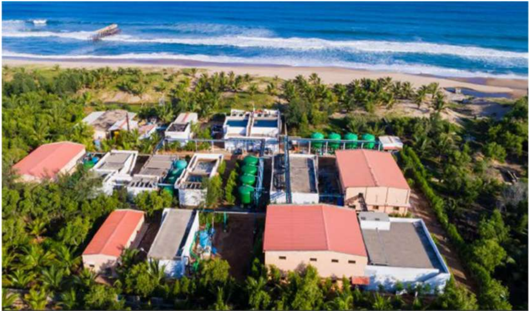
Fig. 2.4 Desalination plant in the Hetero Premises
